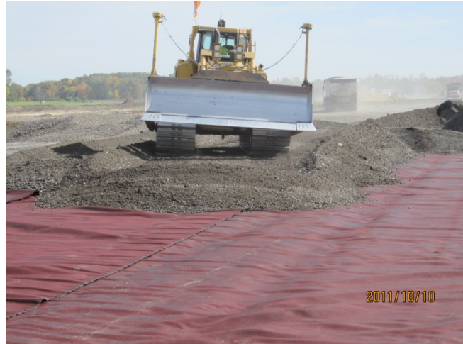
Image 4 – Spreading aggregate over geosynthetic
